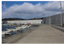
Levee looking from the harbor
