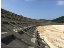
First levee with a height of 7.7m *as of August 2015
